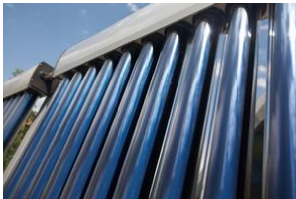
Figure 16: An Evacuated Tube Collector
